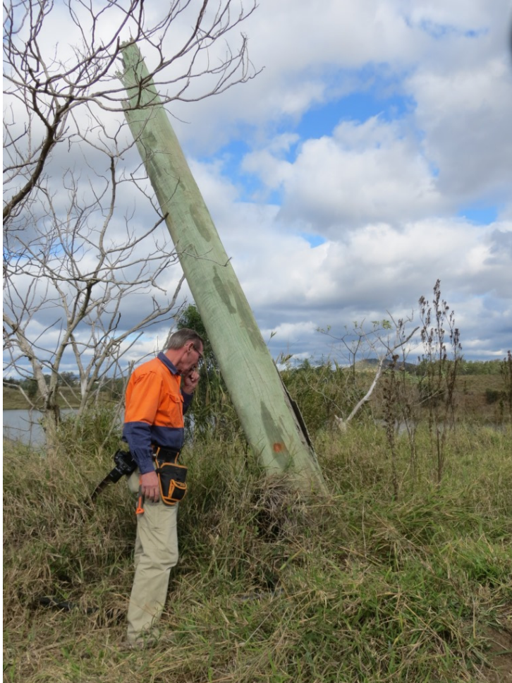
Photo 1 – View of pole from the North. Note paint dot indicating North.
