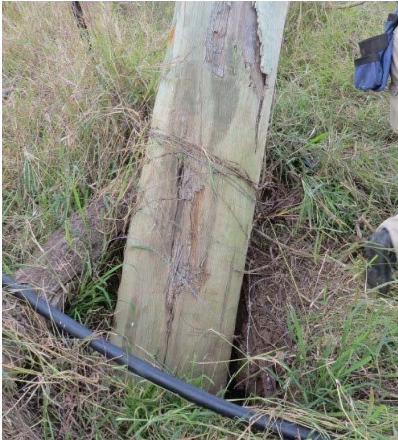
Photo 11 – Scouring at front of post to a depth of approx. 250 mm from actual ground. Note also wire and log debris etc.
