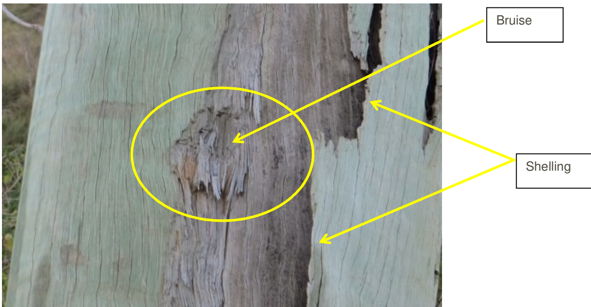
Photo 16 – Close up of bruising damaged middle section of pole and typical shelling
