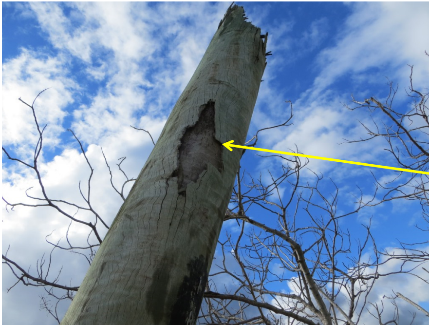
Photo 17 – Damage to upper section of remaining pole. Appears to be shelling
