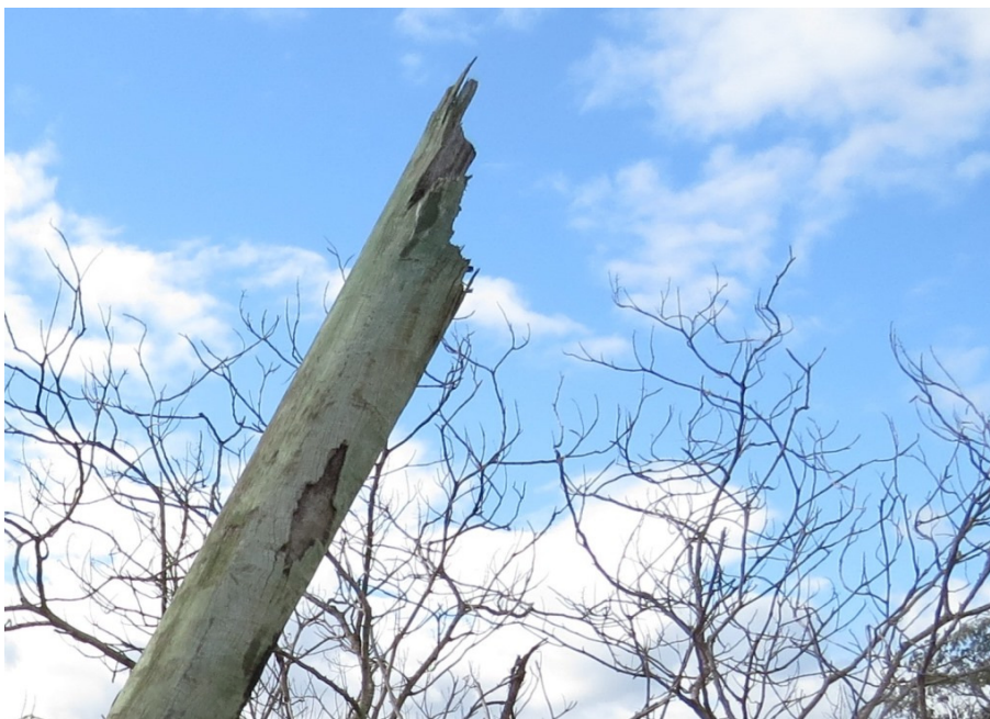
Photo 18 – Pole fracture viewed from the SW
