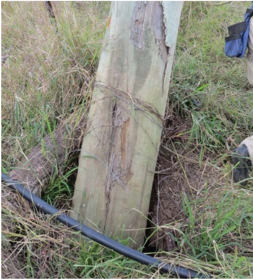
Photo 8 – Debris around base of pole
