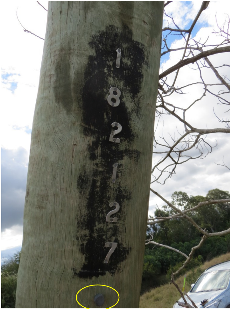
Photo 4 – Pole Identification # and Current leakage test point (highlighted)
