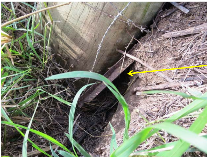
Photo 12 – Scouring to rear (SE) of post to approximately 800 mm from actual ground
