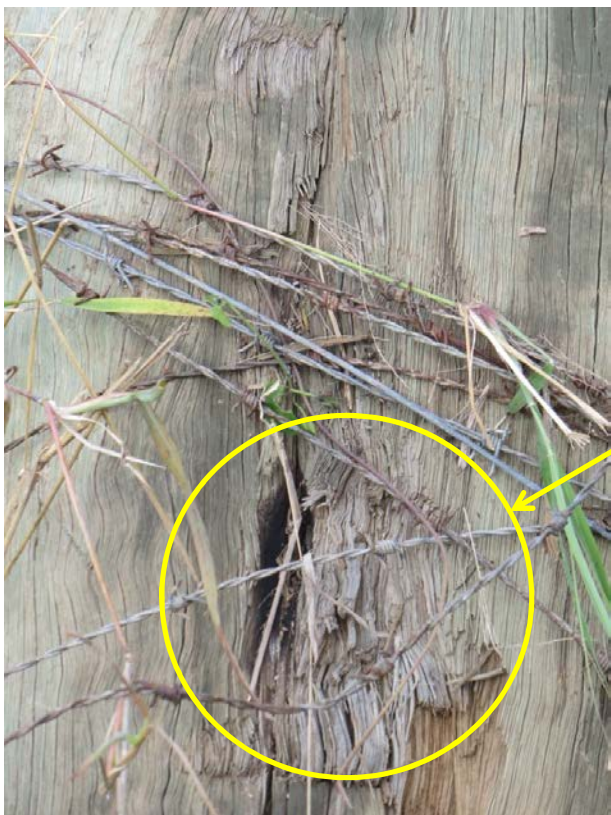
Photo 14 – Close up of damage to lower portion showing bruising
