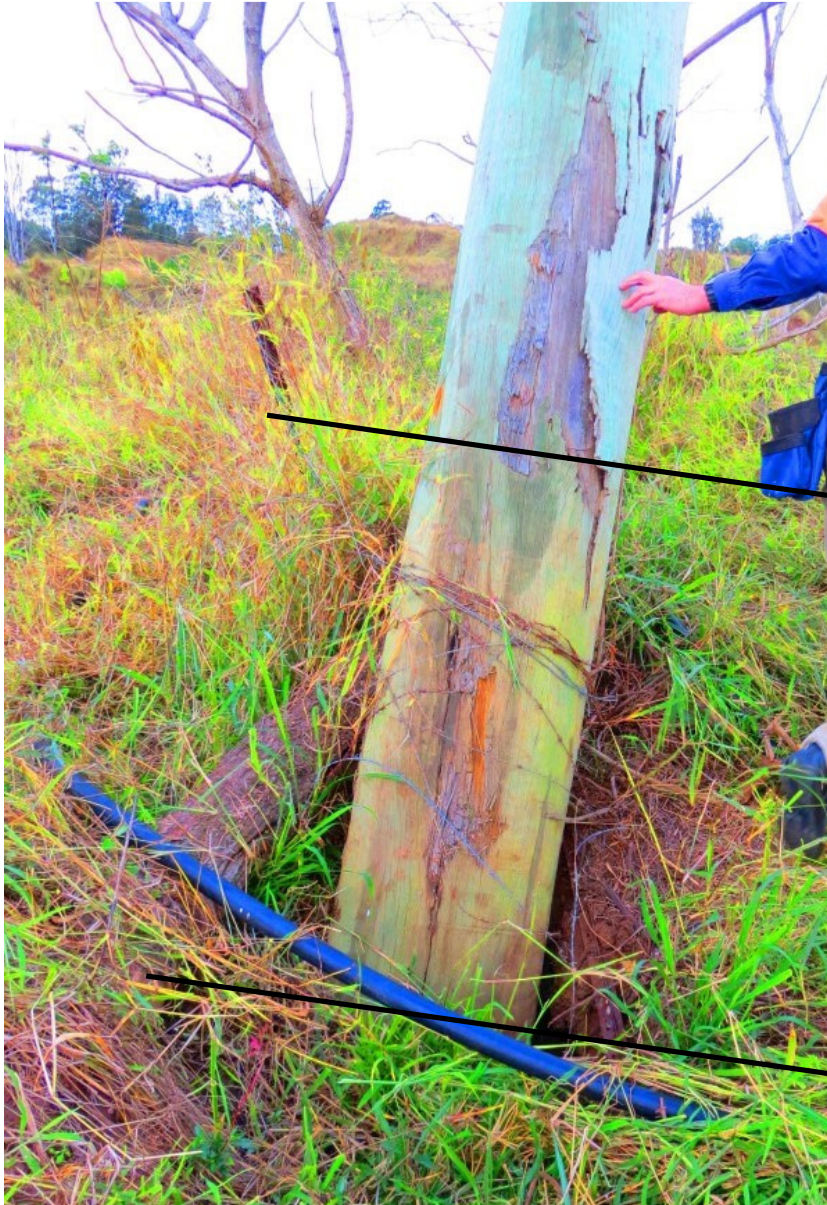
Photo 10 – Digitally enhanced picture of base of pole indicating height of slight colour variation against pole approximately 1100 mm up from ground line.
