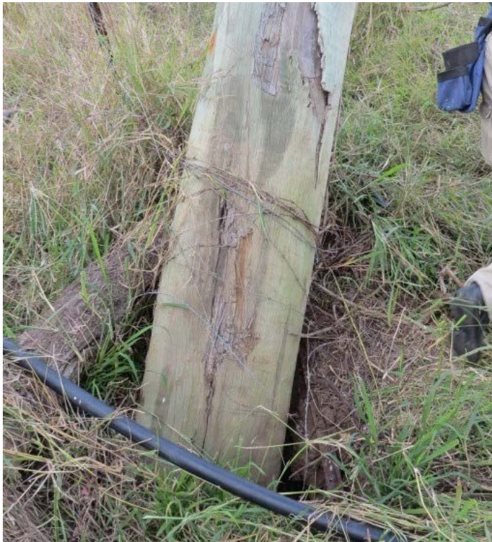
Photo 13 – Damage to lower portion of pole
