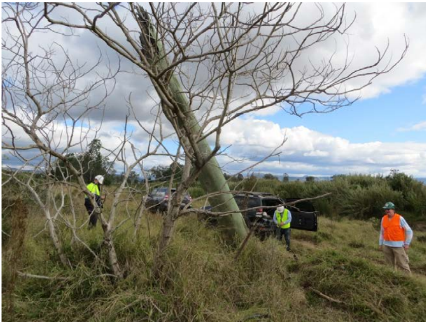
Photo 3 – View of pole from the East
