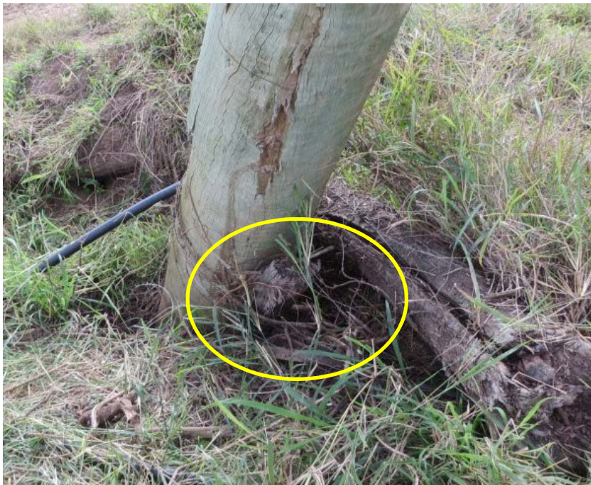
Photo 9 – Evidence of possible top of old fence post adjacent to post
