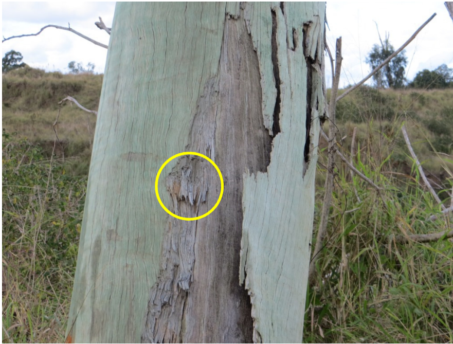
Photo 15 – Damage to middle section of pole
