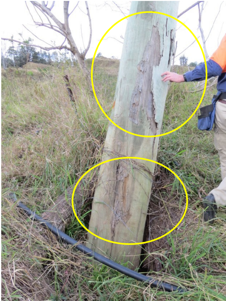
Photo 6 – Bruising/damage to pole on NW face highlighted
