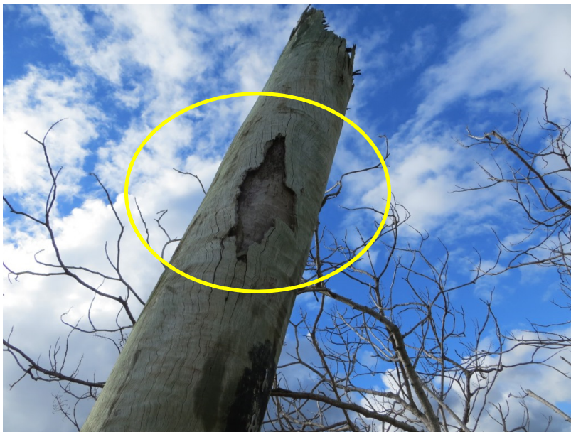
Photo 7 – Damage (possible shelling) to pole on West face highlighted
